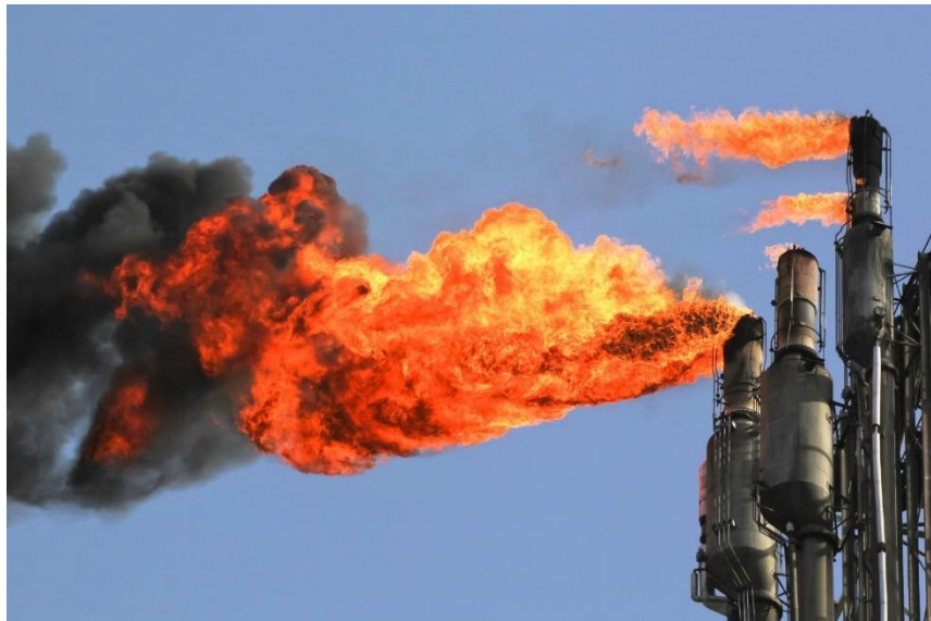
Texas fined industries an average of three pennies per pound for illegal air pollution released during industrial malfunctions and maintenance from 2011-2016, not enough to provide a financial incentive to repair problems or upgrade plants.
